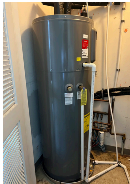
Left to right: Outdoor wall-mounted heat pump units; heat pump water heaters are located in each apartment; the new systems reused existing ductwork, smoothing the transition.
