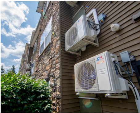
Left to right: Outdoor wall-mounted heat pump units; heat pump water heaters are located in each apartment; the new systems reused existing ductwork, smoothing the transition.
