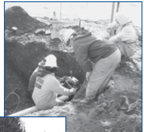
Above: Central Hudson employees work on a gas main extension.
